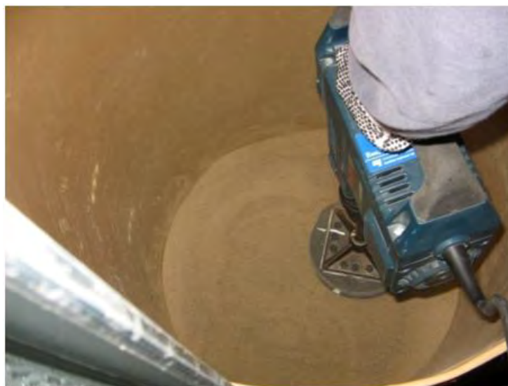
Figure 5-2. Soil compaction in the sand column.
