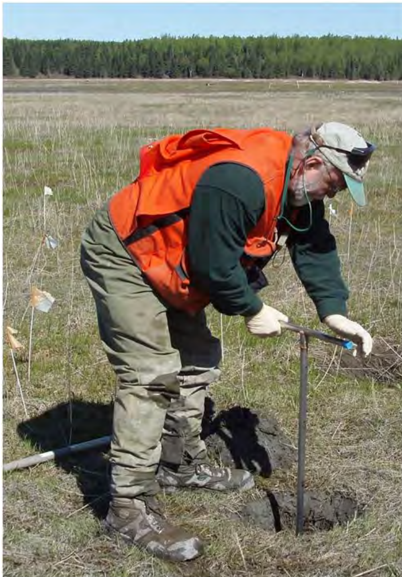
c. Augering the hole for a well.
