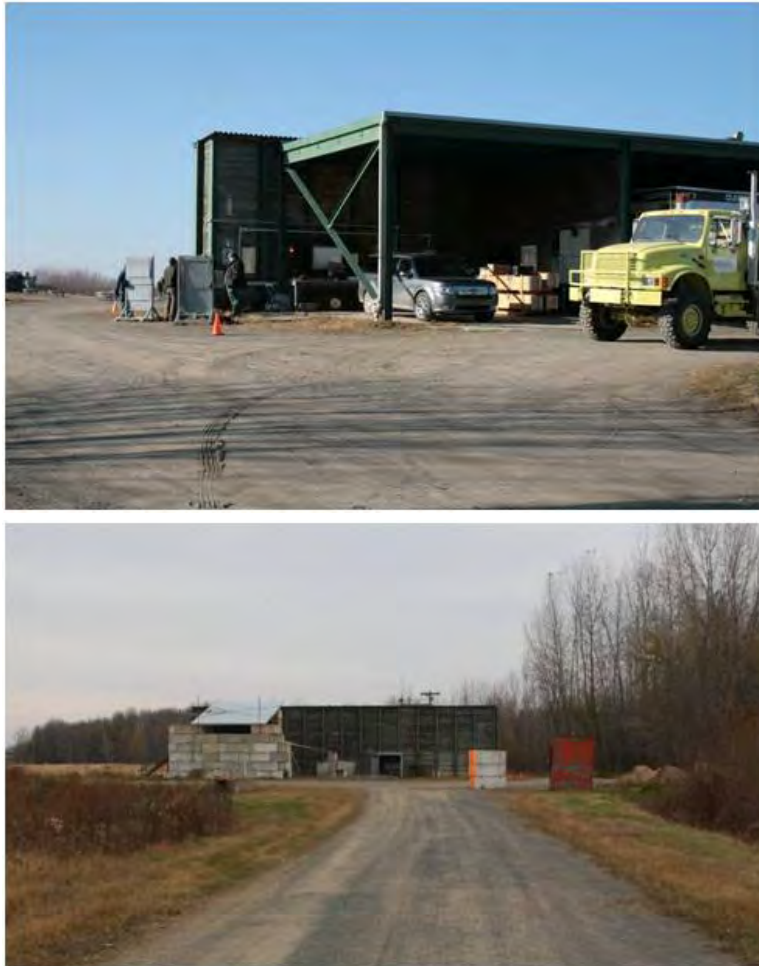
Figure 4-18. Shelter at Batterie 1 and protective wall.
