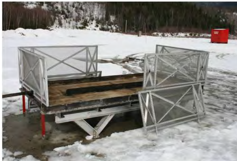
Figure 4-21. Table with new reinforced shields.
