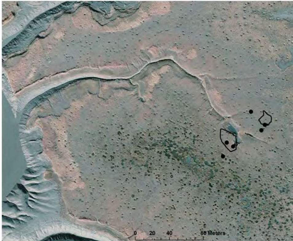
Figure 9-1. Aerial image (Aerometric, October 2010) showing the locations of six shallow groundwater monitoring wells (black dots) at two low-order detonations sites on a salt marsh impact area. The scatter area of the Comp B residues are outlined in black. The craters are located on the south boundary of each outline. Sites are designated LO2 (on the east of the distributary channel) and LO3 (on the west side).
