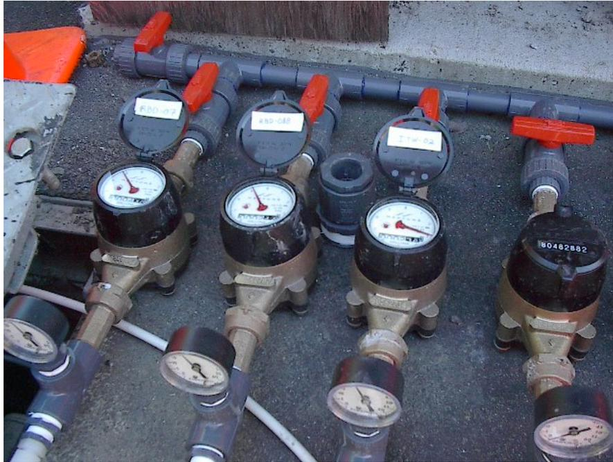
**Figure 3.14** Injection system manifold showing separate control valve and flow totalizer for each injection well.
