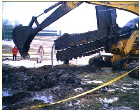
Construction of mulch-filled PRB
