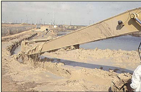
Construction of a bentonite slurry wall vertical barrier
