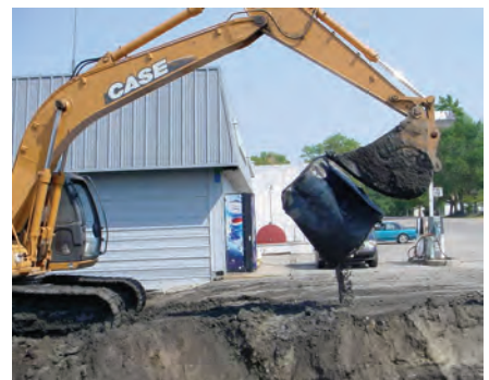
More than 1.5 million storage tanks have been removed from service since 1984 to protect soil and ground water from gasoline contamination. (Photograph courtesy of South Dakota Petroleum Release Compensation Fund.)
