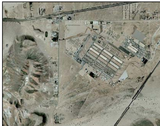
Barstow's Yermo Annex has several designated waste management areas. Photo from Google maps
