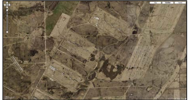
Aerial view of Joliet Army Ammunition Plant. Photo is from Google maps.
