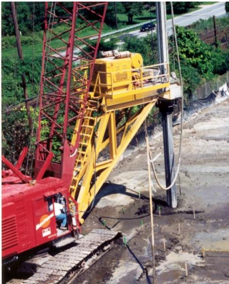
Figure 5.3: A crane-mounted soil-mixing rig
