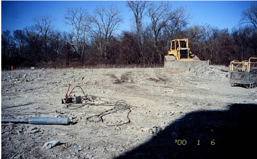
Figure 9.5: Final shaping/contouring of in-situ S/S using a dozer
