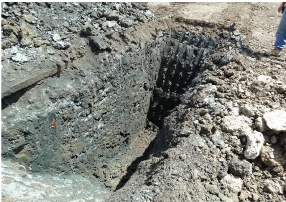
Figure 8.19: Trial pit in an S/S soil monolith
