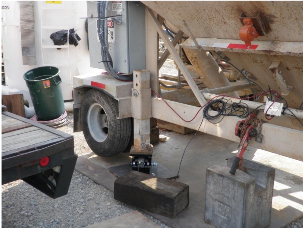
Figure 8.18: Reagent silo electronic scale and calibration weight
