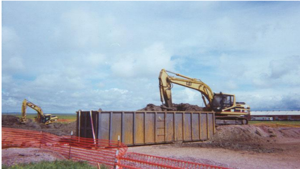
Figure 3.8: Ex-situ treatment in a roll-off box
