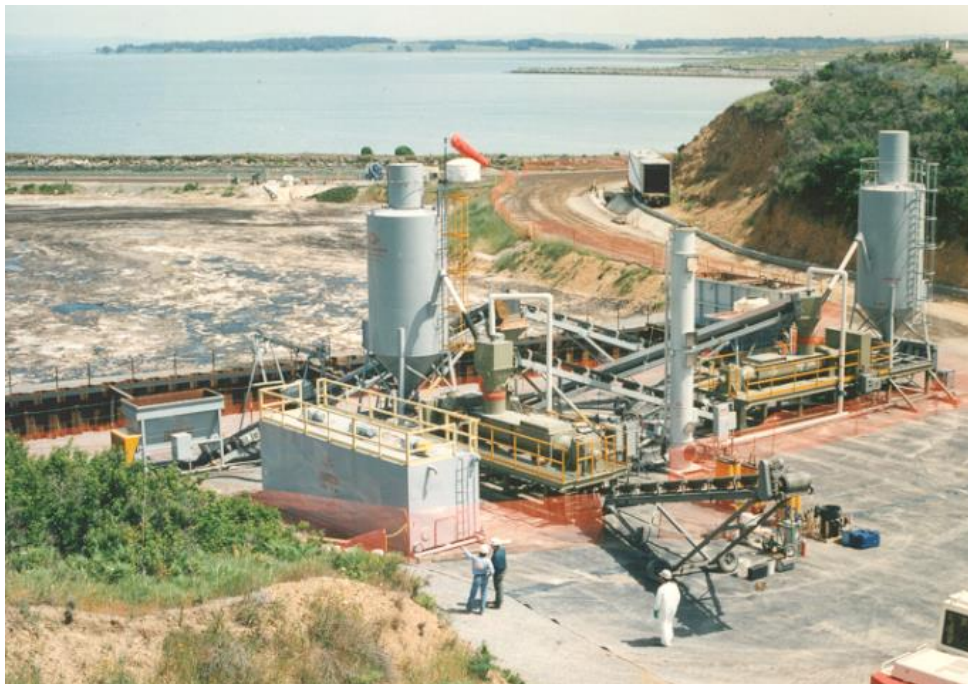
Figure 3.4: Treatment facility to chemically S/S acid sludge tar
