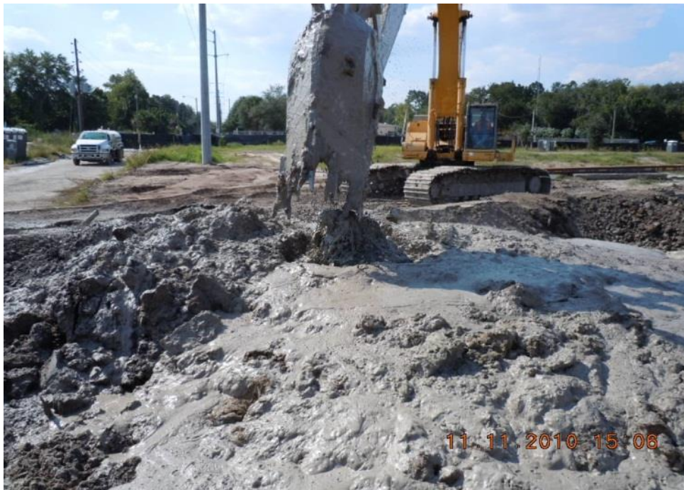
Figure 5.20: Bucket mixing of coal tar soils to depth of 15 ft (5 m)
