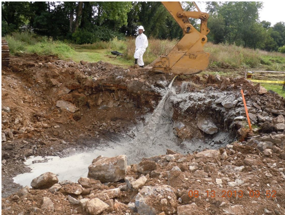
Figure 1.2: Installing a grout slurry blanket to reduce emissions during in-situ S/S treatment
