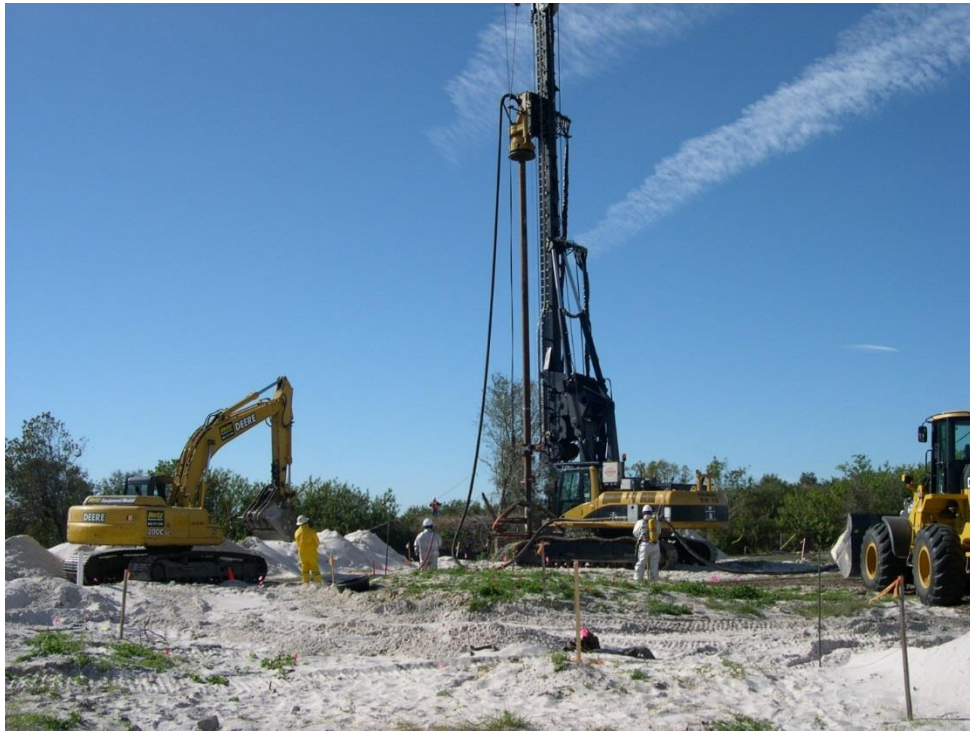
Figure 8.10: Eight-foot (2.5 m) in-situ auger and carrier assembly
