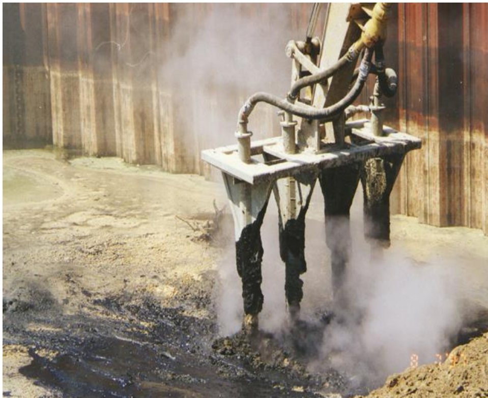
Figure 3.11: In-situ S/S treatment of oily sludge
