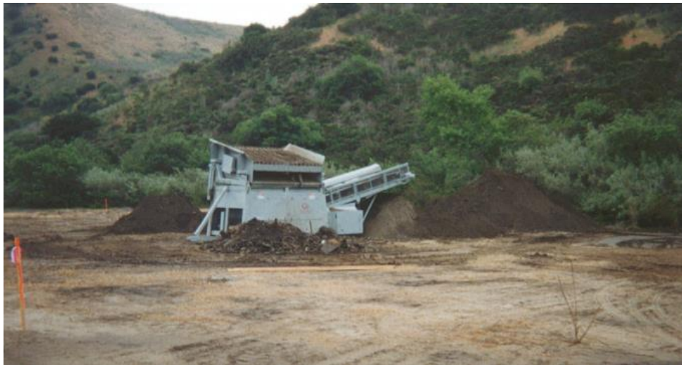
Figure 4.20: Grizzly screen for separation of large debris, with over-sized material, to the left and processed soil for ex-situ mixing, right
