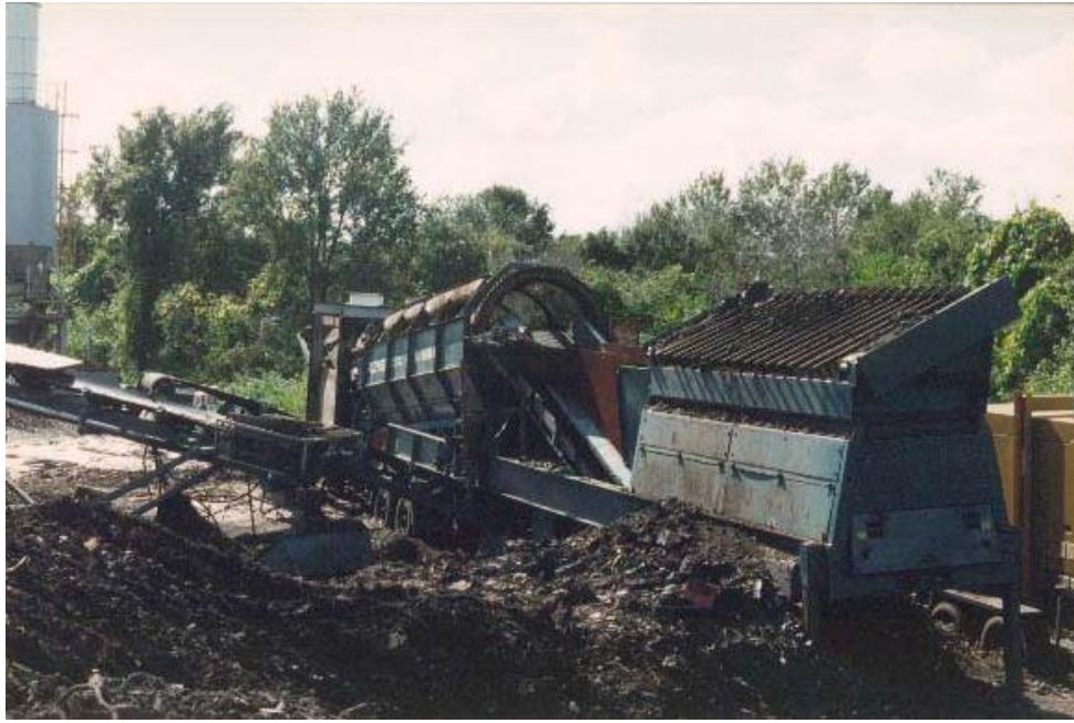
Figure 4.21: Grizzly screen (foreground) combined with a trommel to remove battery casings and debris from excavated material
