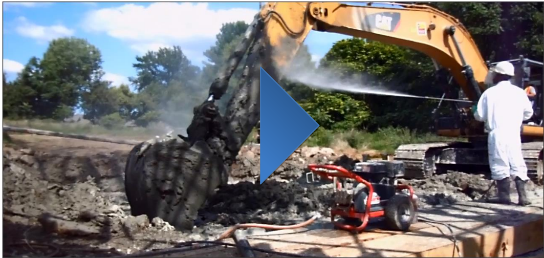
Figure 8.12: Pilot test for in-situ bucket mixing
