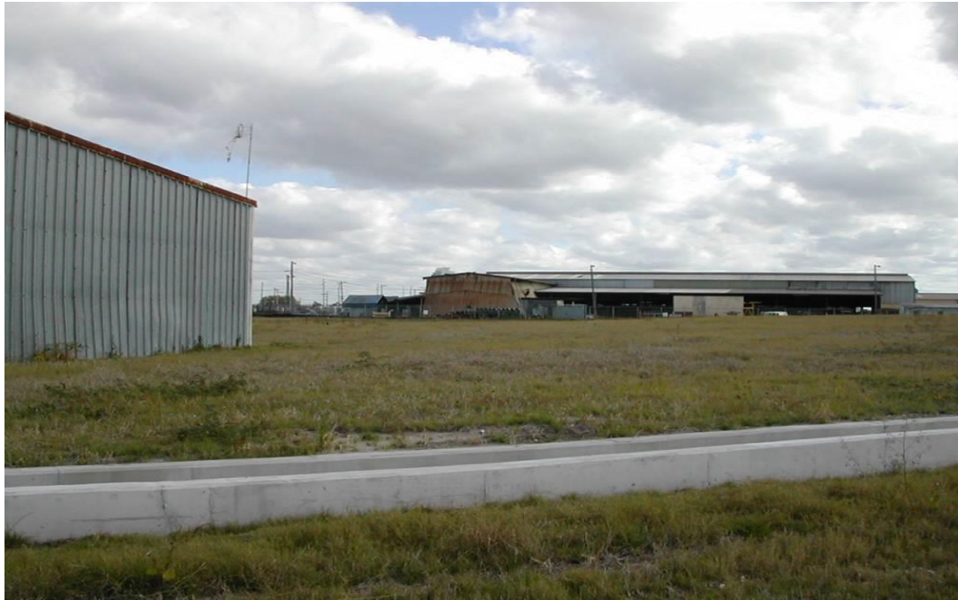
Figure 9.14: GCL and soil cover with drainage channel, Peak Oil Site
