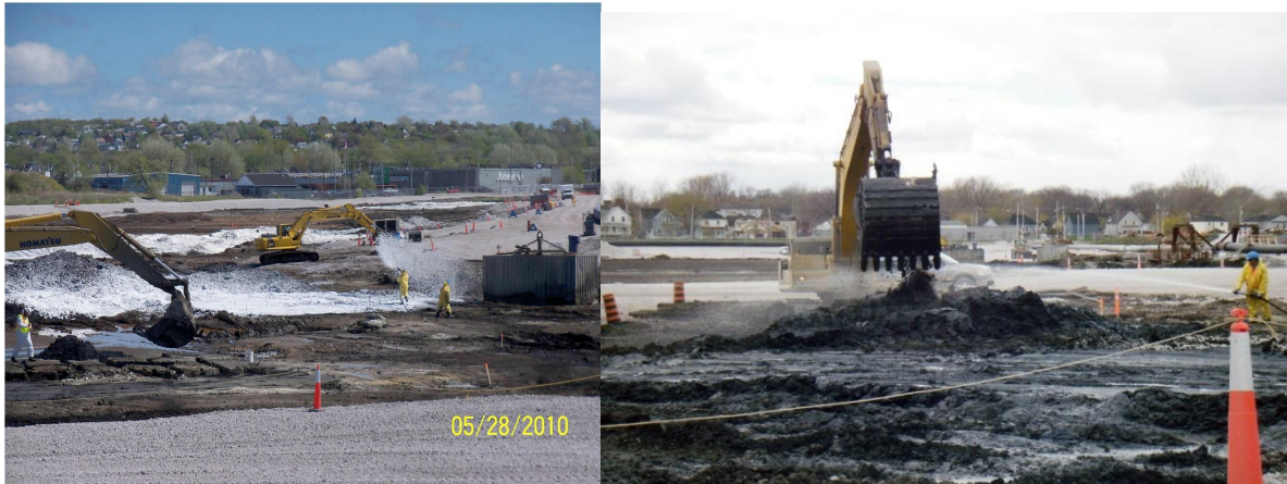
Figure 4: In-situ S/S with dust control conveyance boxes and odour control foam (white) and pressure washer application of bio-solve
