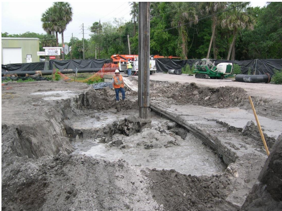
Figure 5.12: In-situ treatment of soil under a live fibre optic line
