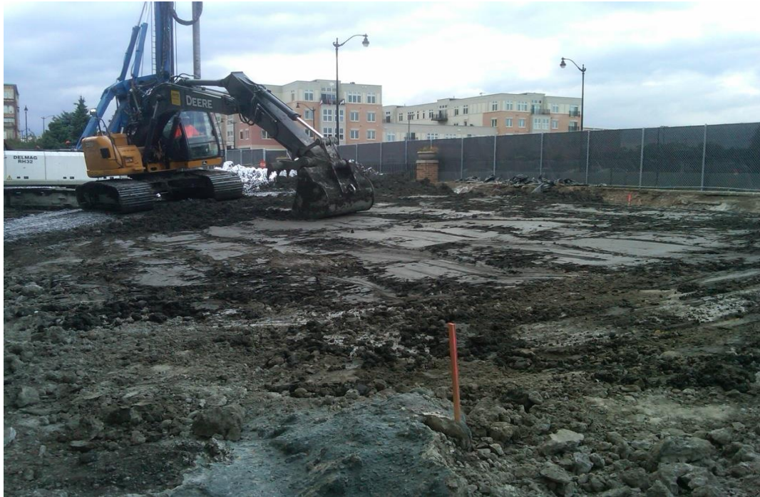
Figure 9.4: Direct placement of S/S swell by an excavator for final grading
