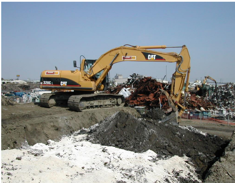
Figure 4.18: Bucket mixing hydrated lime and oily waste in earthen pit
