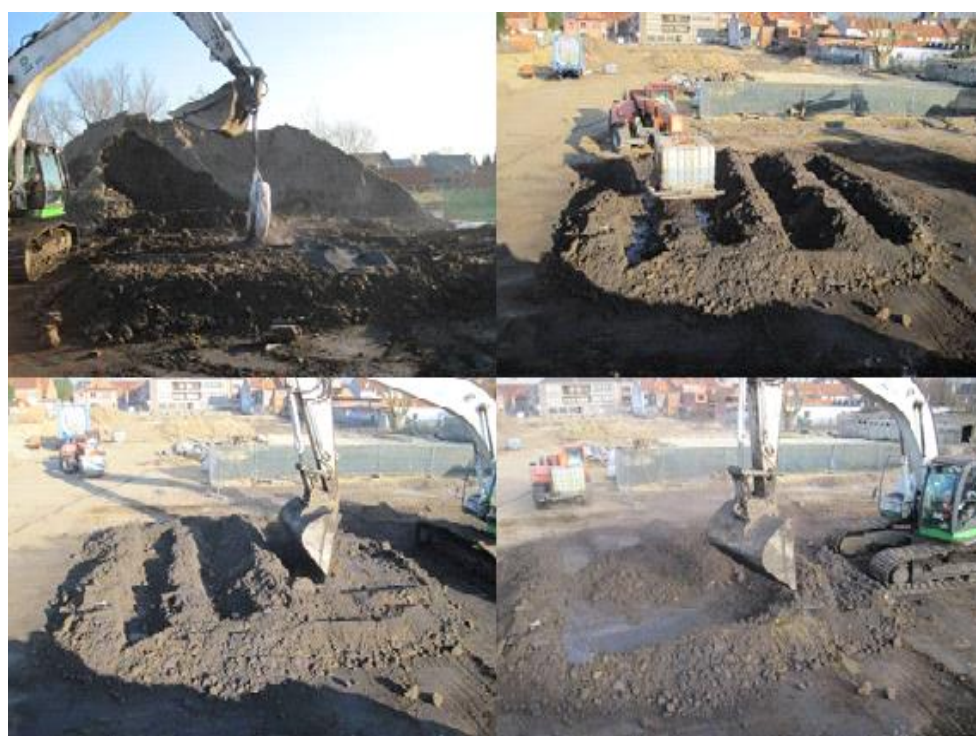
Figure 3.1 Lead-contaminated soil and battery casings from a former battery-recycling site, subsequently chemically stabilized
