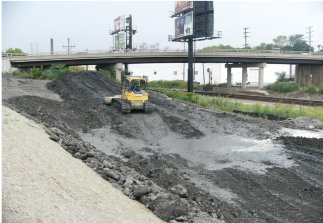
Figure 9.6: Reconditioning and placement of in-situ S/S swell
