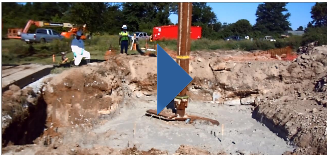
Figure 8.11: Pilot test using a 10 ft (3 m) diameter in-situ auger
