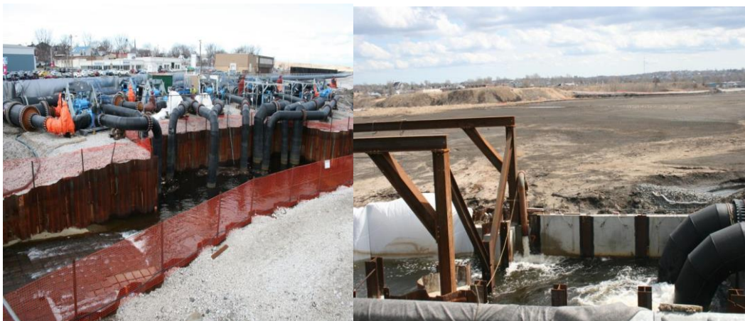
Figure 3: South Tar Pond Dewatering
