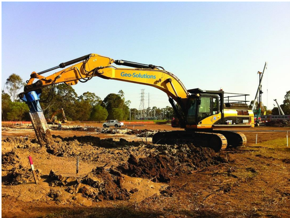
Figure 5.14: Backhoe (excavator) Operated Soil Stabilizer (BOSS)
