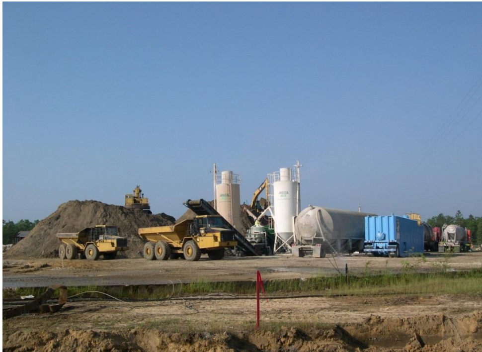
Figure 8.13: Ex-situ pug-mill with support equipment
