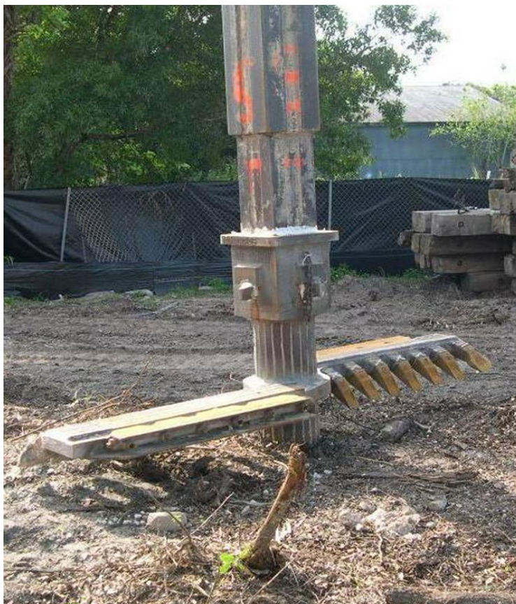
Figure 5.7: Auger used at a coal gas plant site in FL
