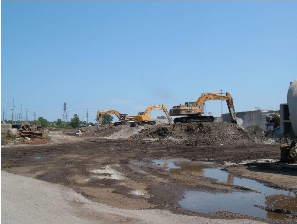
Figure 4.17: Excavator mixing of Portland cement into Pb-contaminated soil and debris
