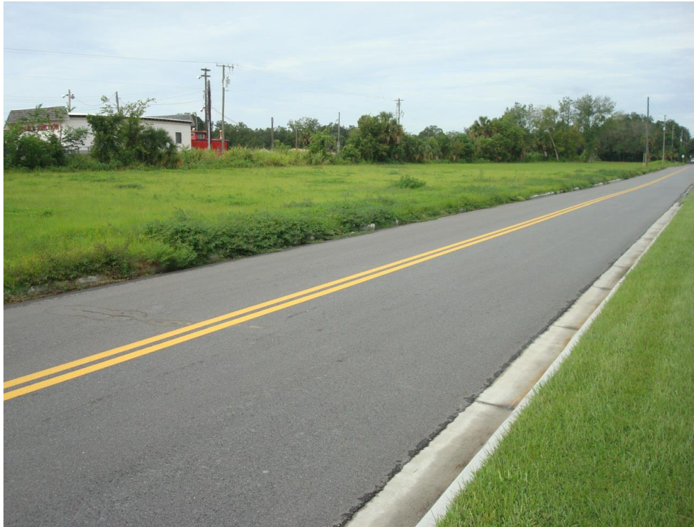
Figure 9.21: Reconstruction of an asphalt roadway over an S/S monolith in Sanford, FL
