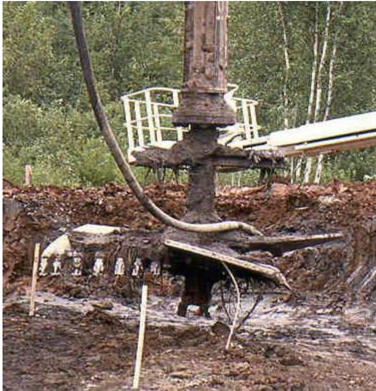
Figure 5.6: Auger used at the USX Site, Duluth, MN
