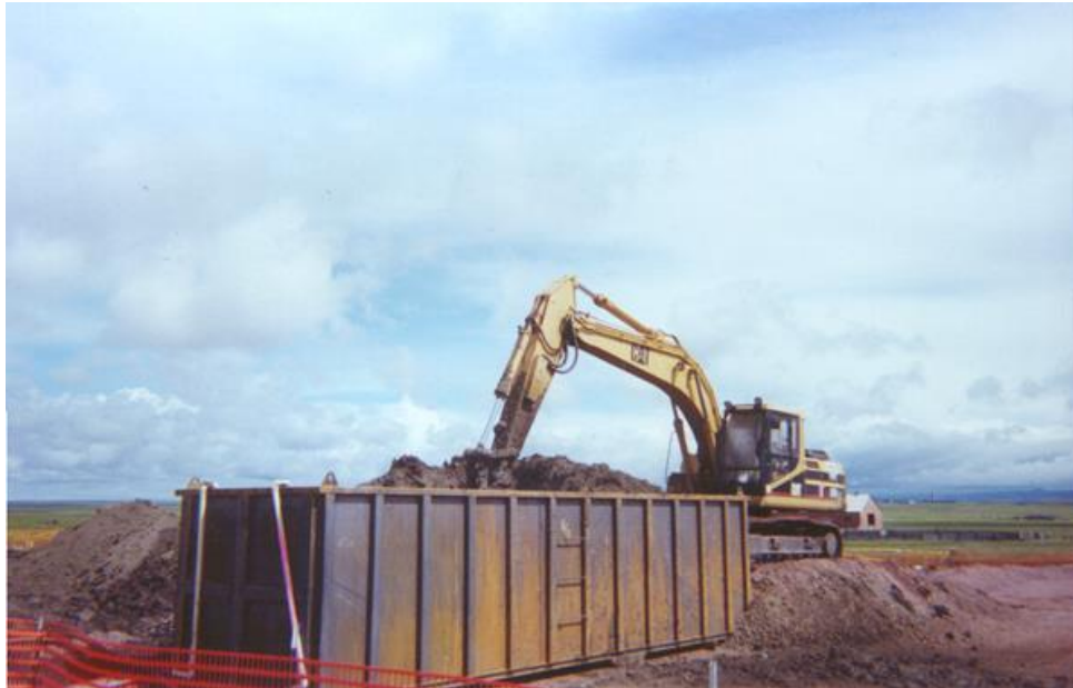
Figure 4.19: Stabilization of hexavalent chromium-contaminated soil in a roll-off box
