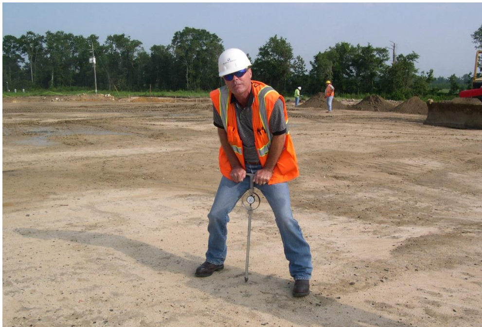
Figure 6.16: Using a field penetrometer to assess strength of field placed S/S material
