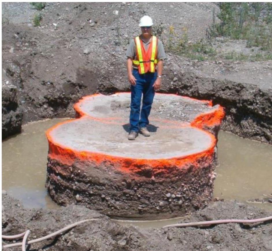
Figure 5.11: showing typical excavated overlapping columns
