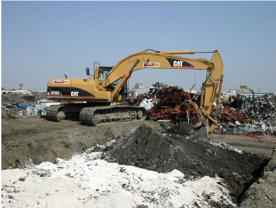
Figure 8.1: Hydrated lime added to waste in a mix pit
