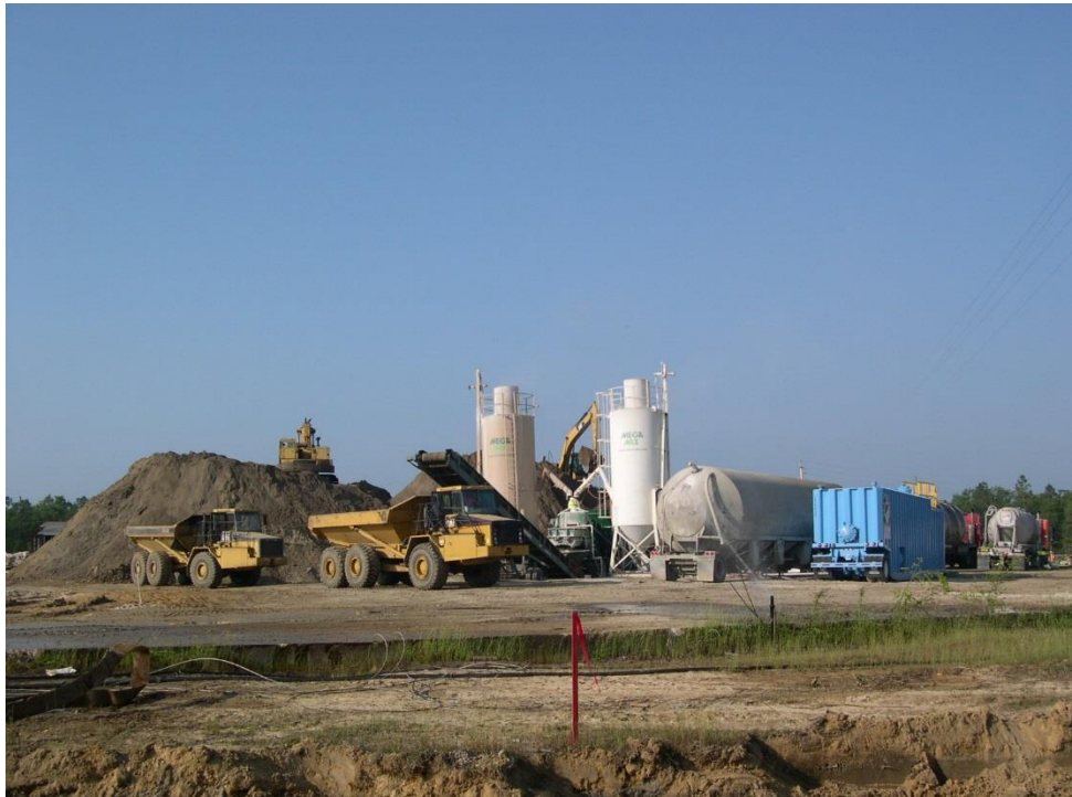
Figure 3.9: Typical ex-situ S/S equipment, including pug-mill, silos, reagent tank, water tank, stacker and haulage
