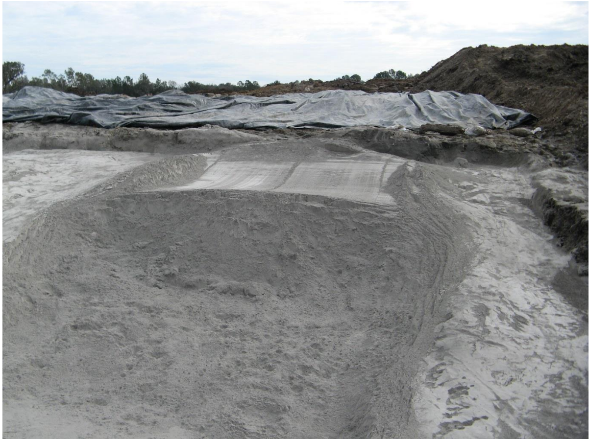
Figure 8.2: Fly ash stockpile on a treatment site with its cover removed
