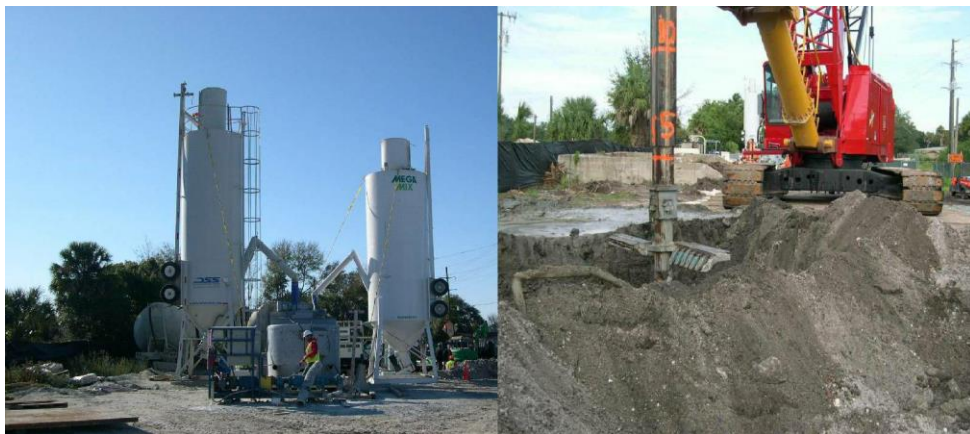
Figure 3.13: Typical in-situ S/S equipment: batch plant with reagent silos and mix tanks; crane, Kelly bar, and auger
