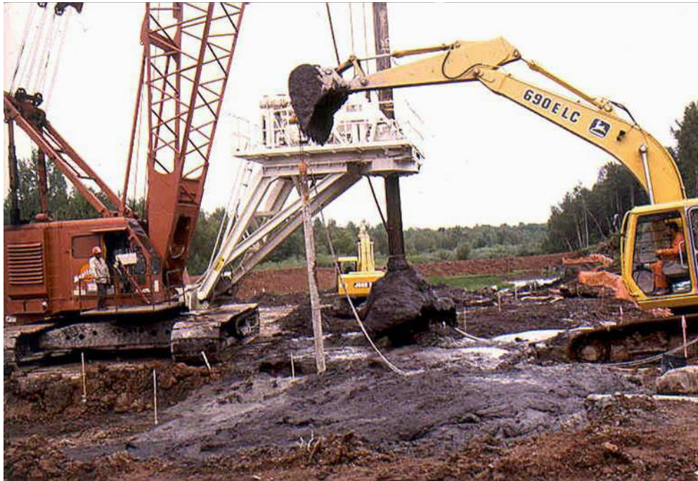
Figure 6.4: Collection of sample using piston tube inserted by excavator,
