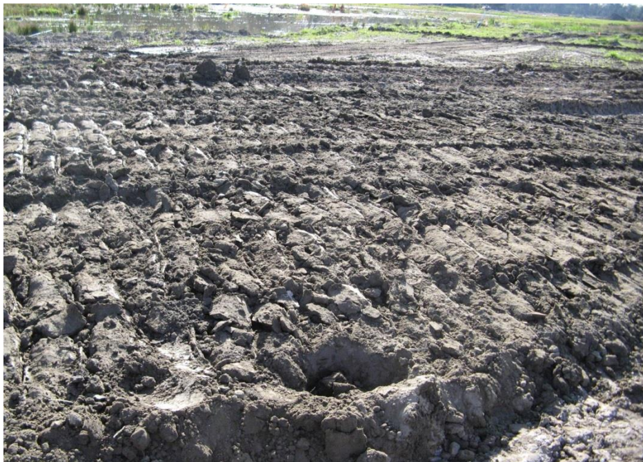
Figure 4.24: Placed ex-situ S/S-treated material after multiple passes of the dozer
