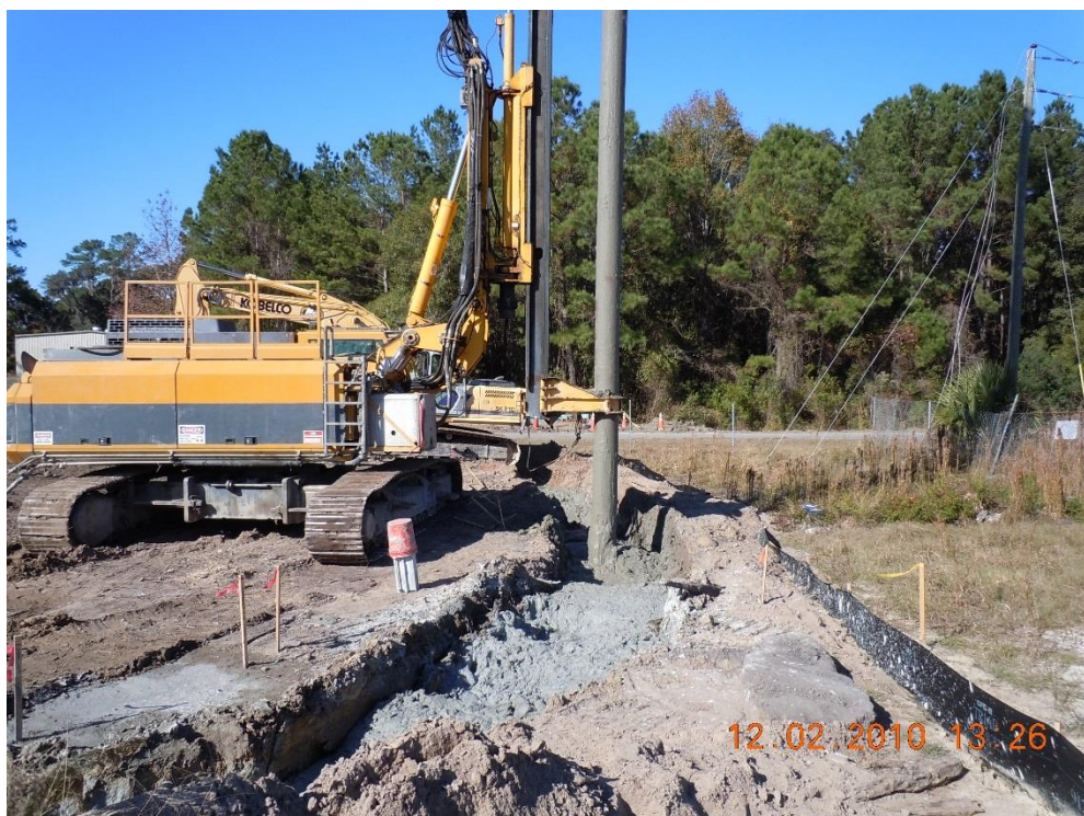
Figure 7.6: Constructing a vertical wall using a Bauer Panel Cutter, Brunswick
