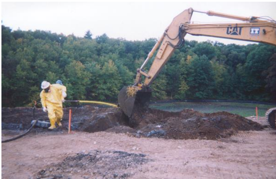
Figure 3.2: Chromium paint pigment-contaminated soil being chemically stabilized in-situ
