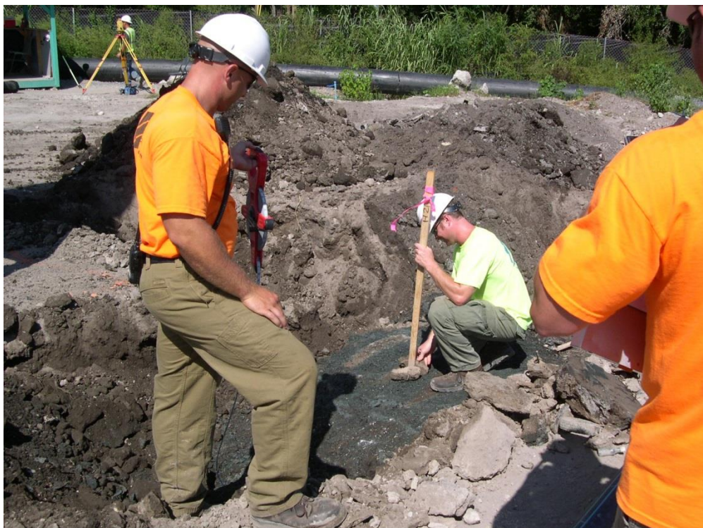
Figure 6.17: Excavating top of in-situ column
