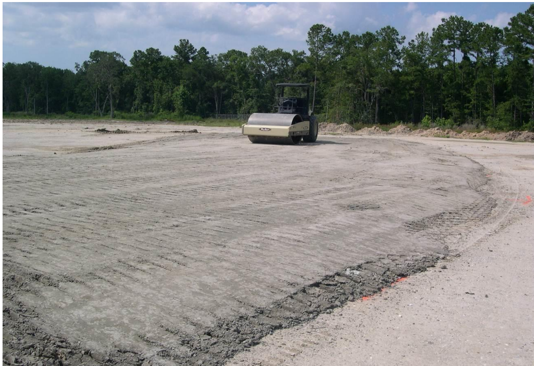
Figure 9.3: A smooth roller being used to compact ex-situ treated material
