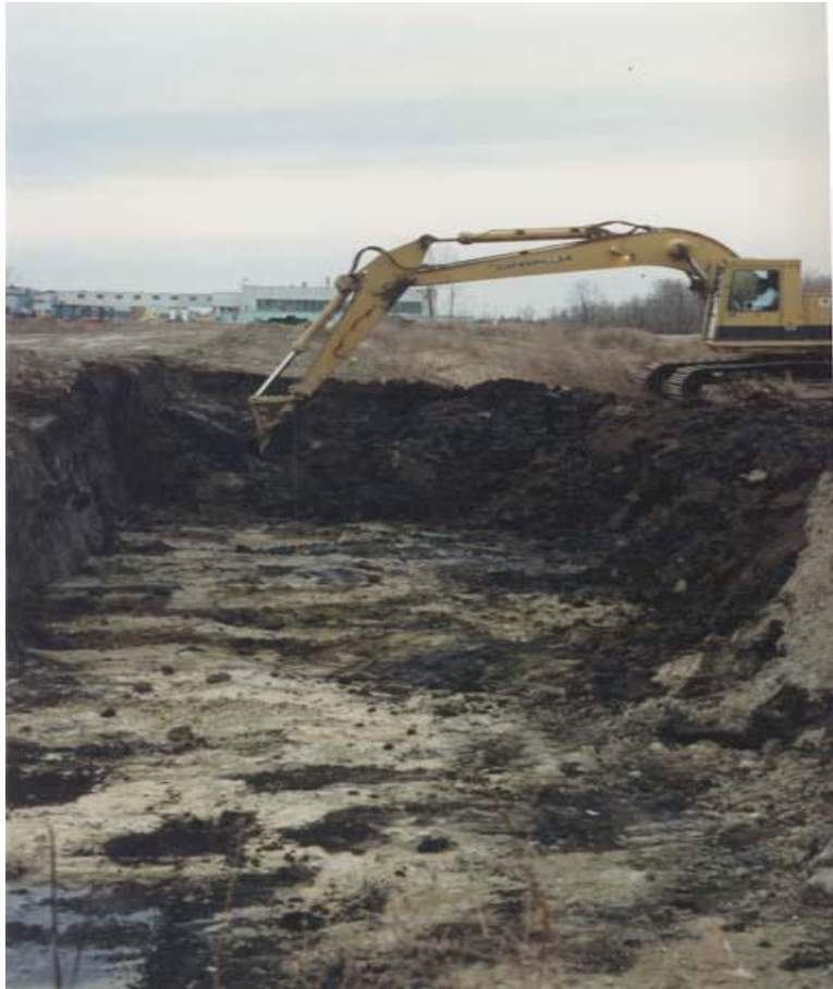
Figure 3.3: A contaminated wastewater sludge being excavated
