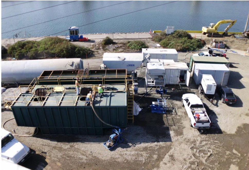
Figure 5.18: A batching plant for a large S/S project
