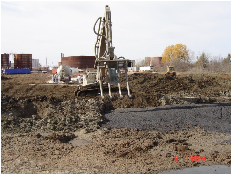
Figure 4.13: Rotating rake mixing attachment
