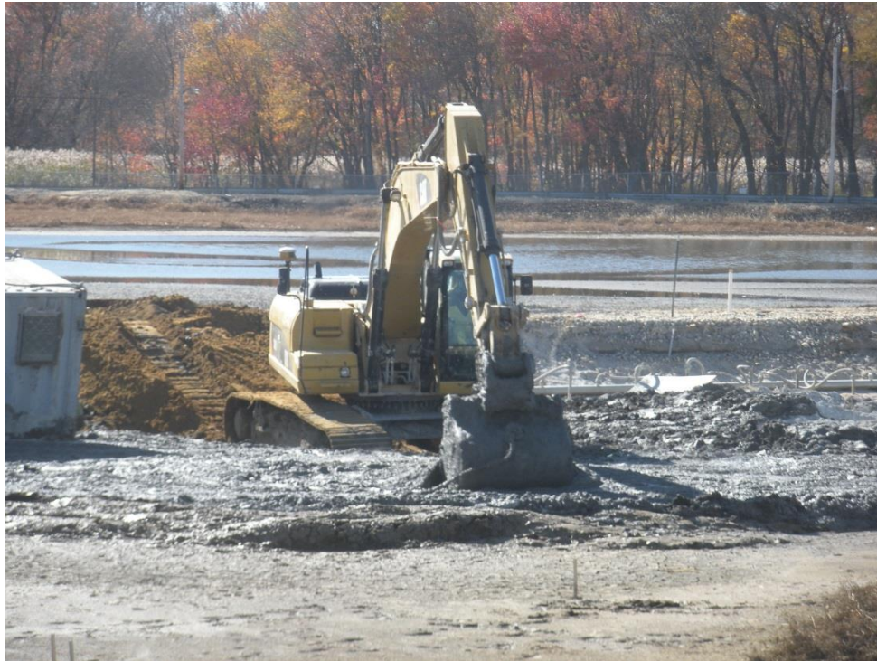
Figure 3.12: In-situ mixing equipment operating on top of S/S treated material
