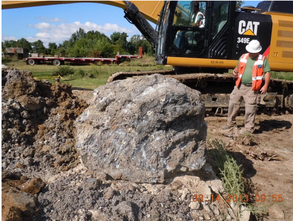
Figure 3.14: A 3 ft limestone boulder excavated to facilitate in-situ treatment
