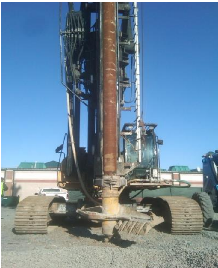
Figure 5.4: An excavator-mounted rig
