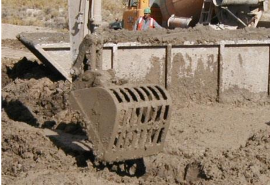
Figure 5.19: Example of bucket mixing
