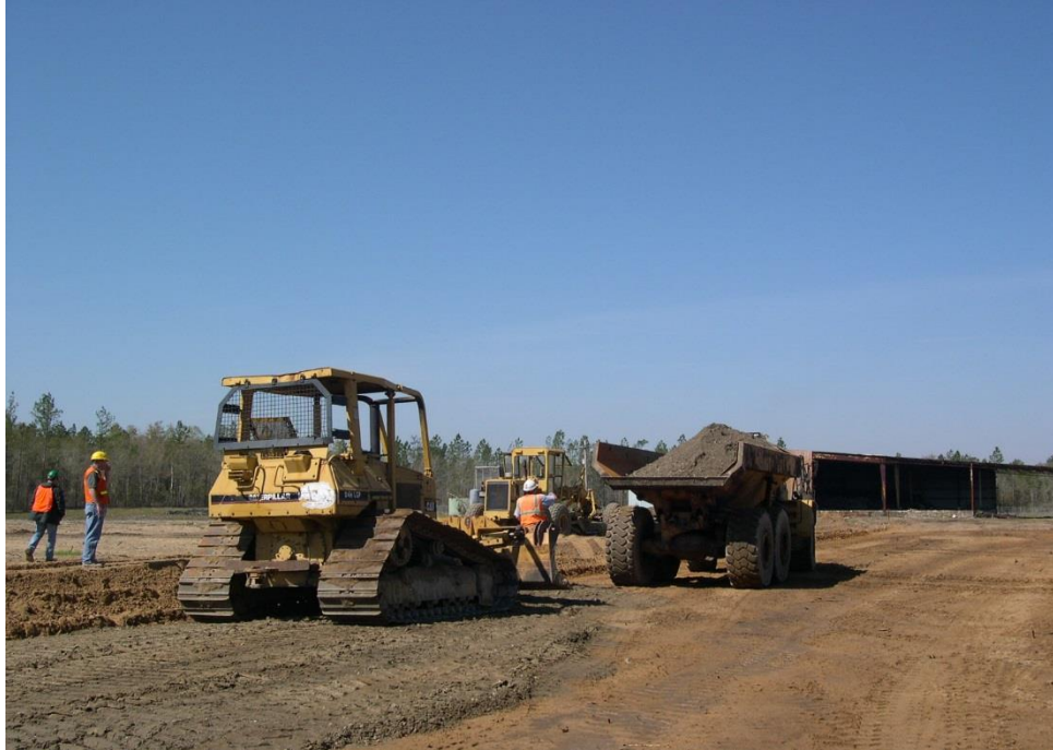
Figure 4.23: Transport and placement of ex-situ S/S material
