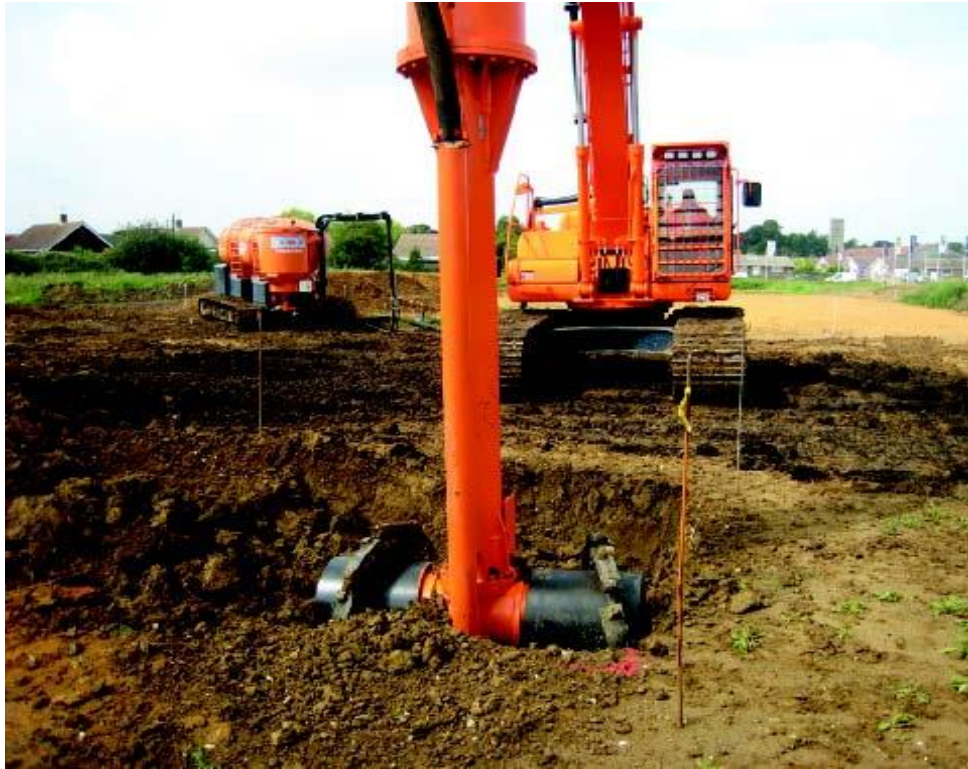
Figure 4.11: Allu PMX Power Mixer™ attachment
