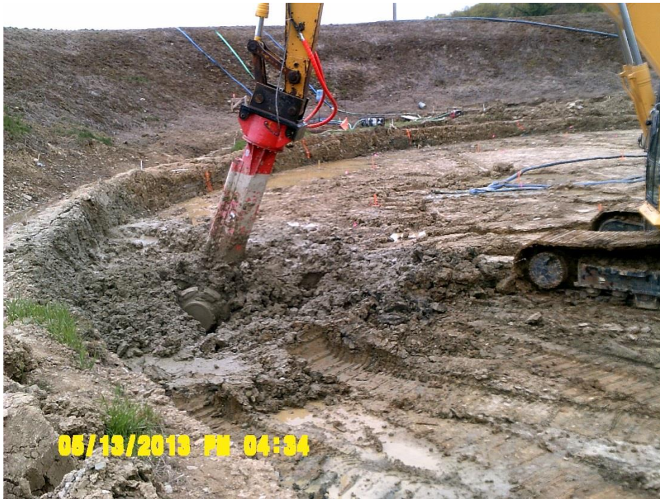
Figure 5.15: Backhoe (excavator) operated soil stabilizer
