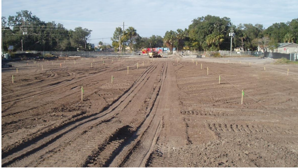
Figure 9.20: A coarse-grained soil-based ET cap over an S/S monolith
