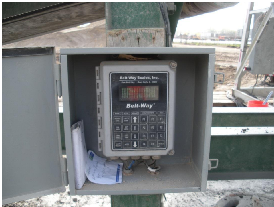
Figure 4.7: Control panel for waste feed conveyor
