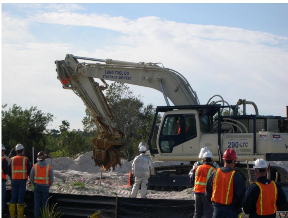
Figure 5.16 Lang mixer- excavator, arm, and mixing head as one unit
