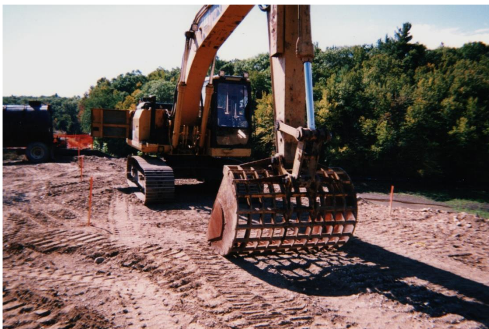
Figure 4.10: Modified excavator bucket for improved mixing
