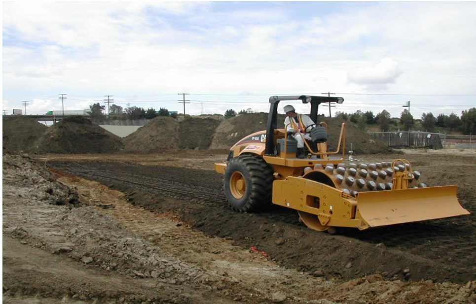
Figure 4.26: Sheep-foot roller compacting S/S treated material (note the oval pads on the roller)
