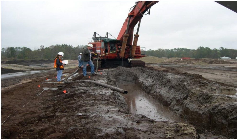
Figure 7.4: Installing a slurry wall, Whitehouse, Florida
