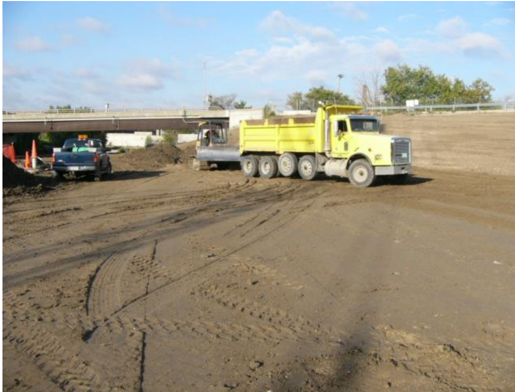
Figure 9.9: Construction of a low permeability clay cap
