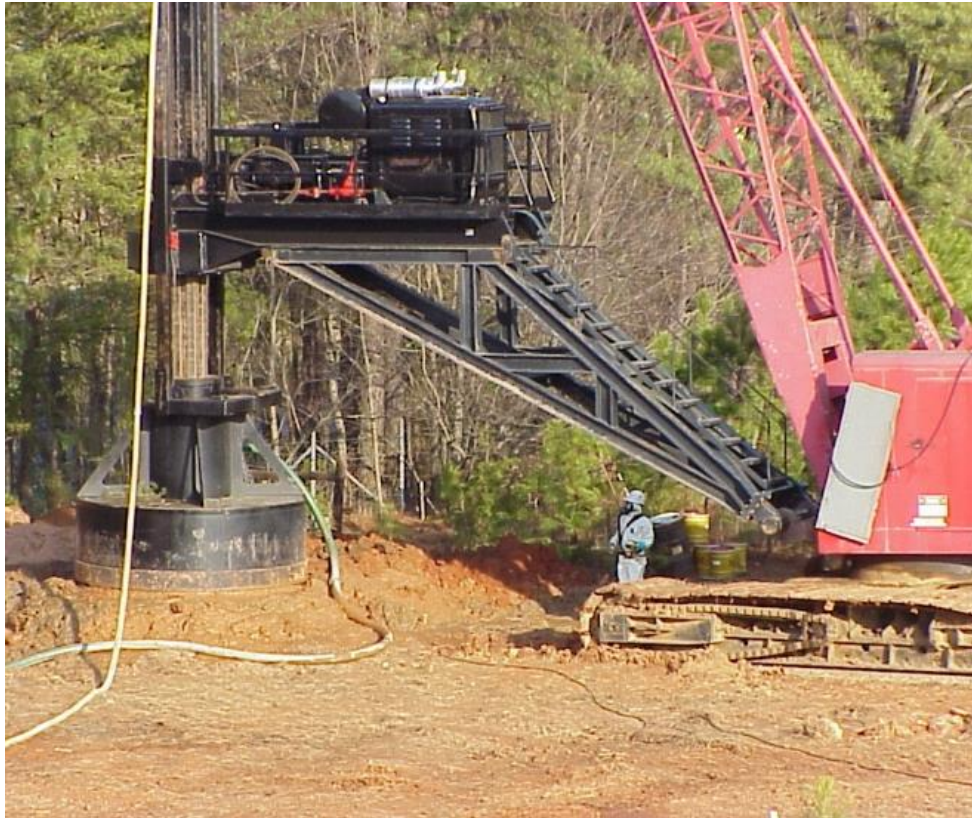
Figure 5.2: A crane-mounted soil-mixing rig
