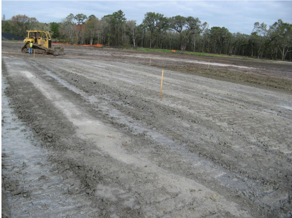
Figure 7.5: Constructing a S/S sub-cap, Brunswick
