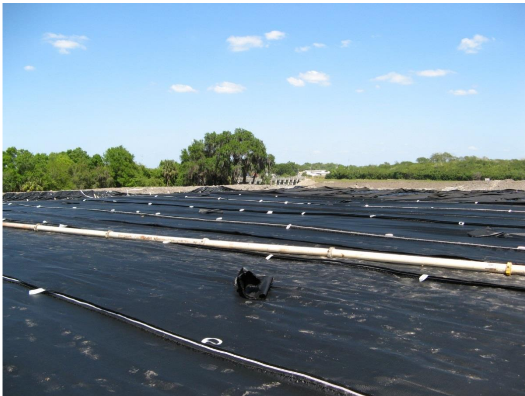
Figure 9.11: Installation of a geo-membrane showing the welded seams between sheets
