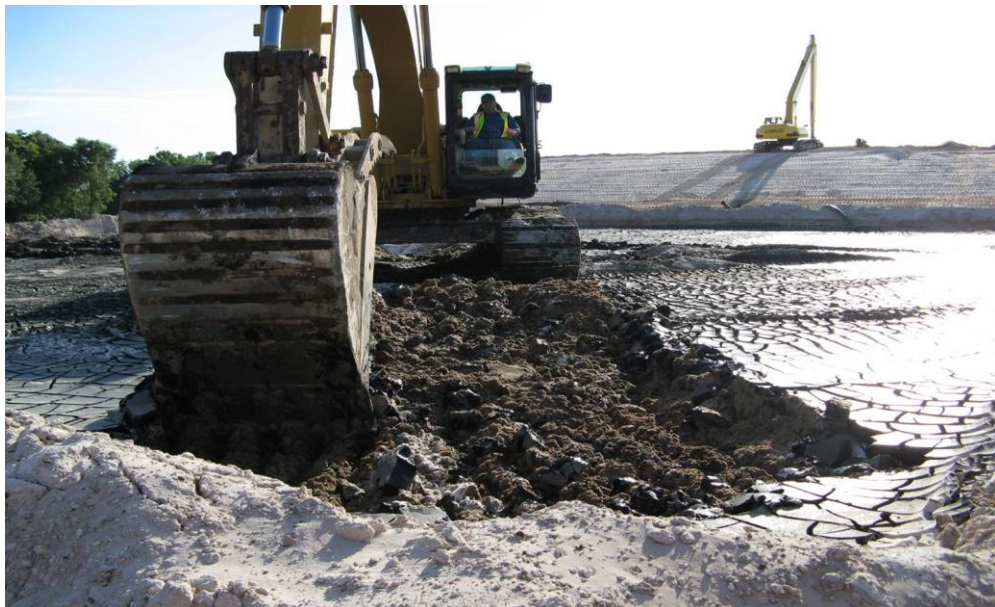
Figure 7.8: Solidifying oily water emulsion Stauffer
