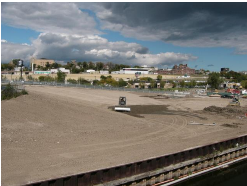
Figure 9.10: Final grading to direct surface drainage
