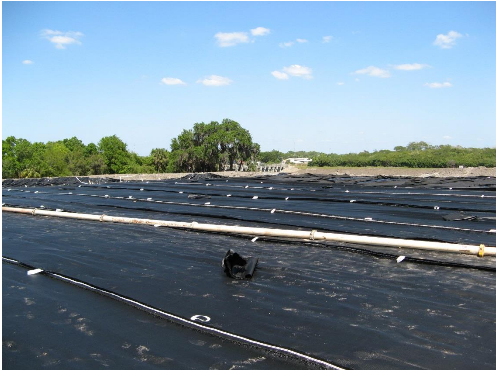
Figure 7.9: Installing an FML at Stauffer
