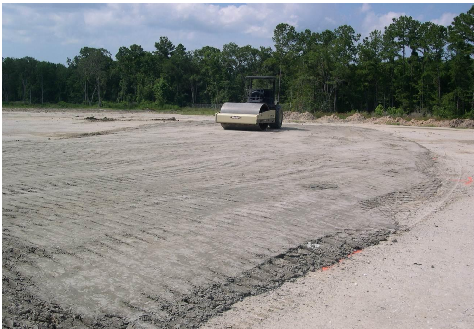
Figure 4.27: Smooth roller compacting ex-situ S/S treated material
