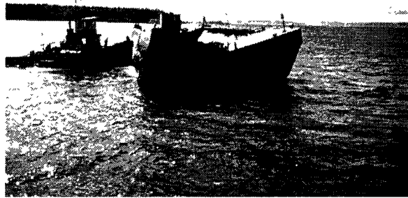
Figure 10. Spreading technique for capping by barge movement at Denny Way, Puget Sound.
